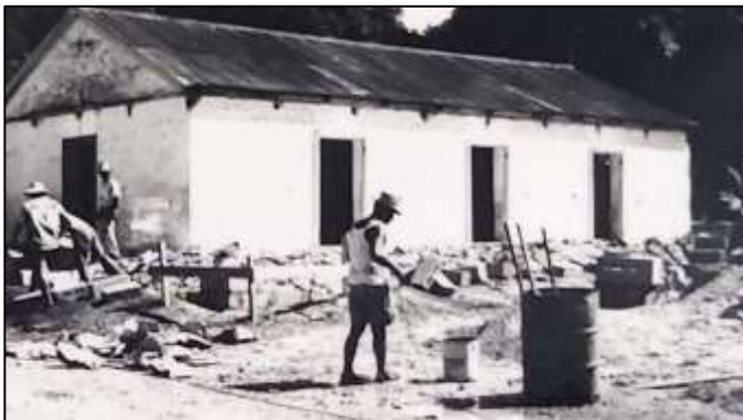
TE KAPUAANGA from another time era, construction of extension on seaside. Year taken and by whom are unknown. Source: National Archives, Avarua.
