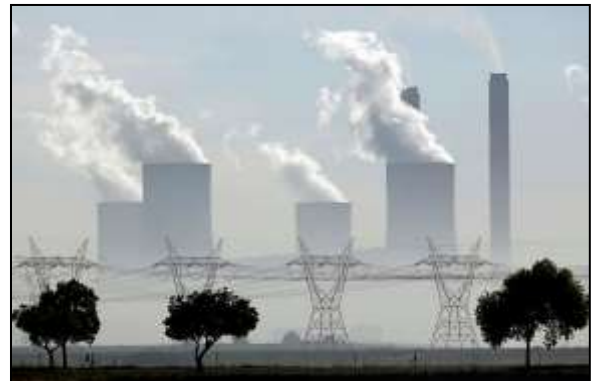
Smoke billows from the chimneys at the coal-fired Lethabo power station in Vereeniging, South Africa, in 2018. (Themba Hadebe/AP)
