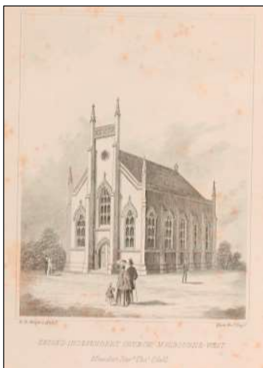
The Avarua Church was based on plans for the Second Congregational Church, Little Lonsdale street, Melbourne (from The Illustrated Australian Magazine, March 1851).
