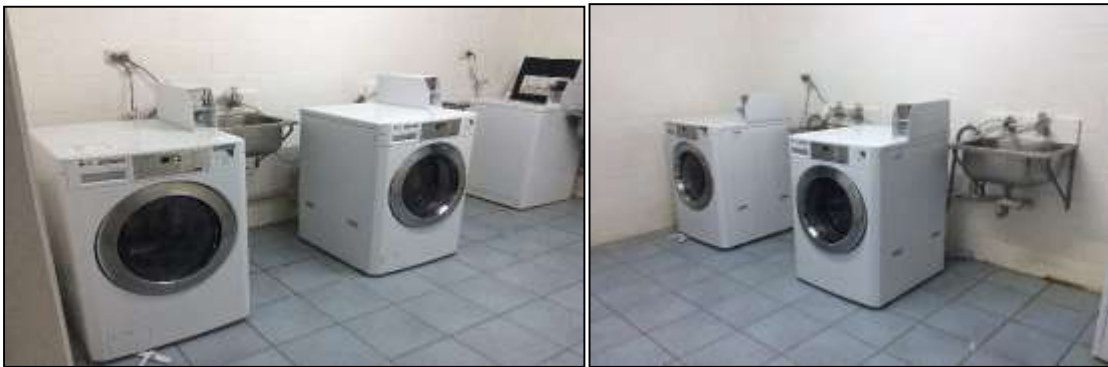
The two new washing machines situated in the Laundry room
