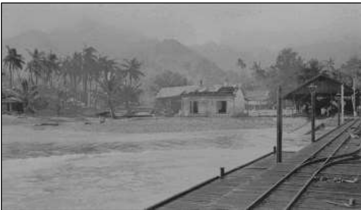
Avarua Wharf from the north. Ravaged roof most likely caused by cyclone. 2 nd colour photo below (from Google) shows Trader Jack's Restaurant and Bar on the same spot as the damaged building above.
