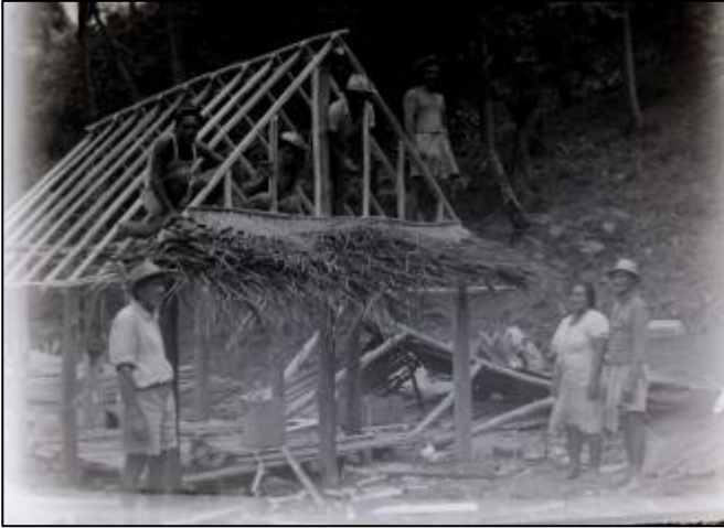
Moe family making a new house up at Takuvaine valley.
