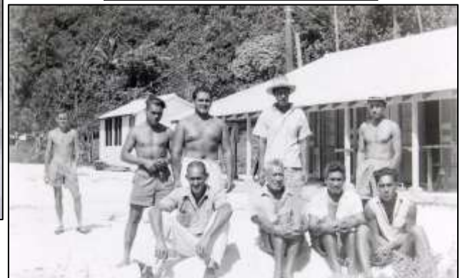
Carpenters who worked on the DSIR Observatory station at Takuvaine Valley
