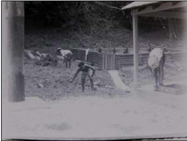
Garden fence completed and cleaning up.
