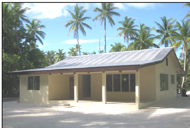
New 2-bedroom CICC Mission House, Palmerston Island
