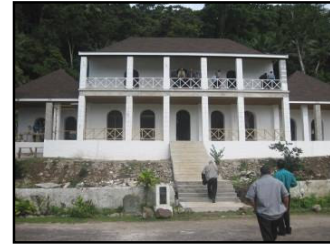
Mission House being renovated as the new CICC head office admin
